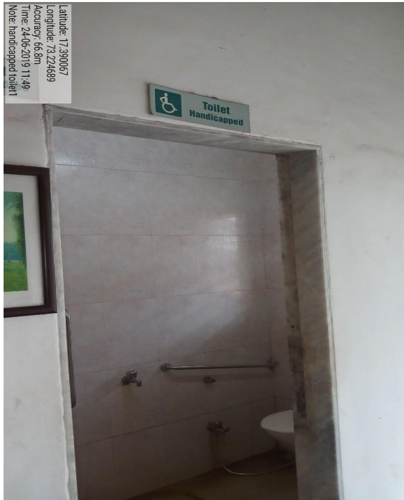
Special toilet for Handicapped students / staff with handle for support
