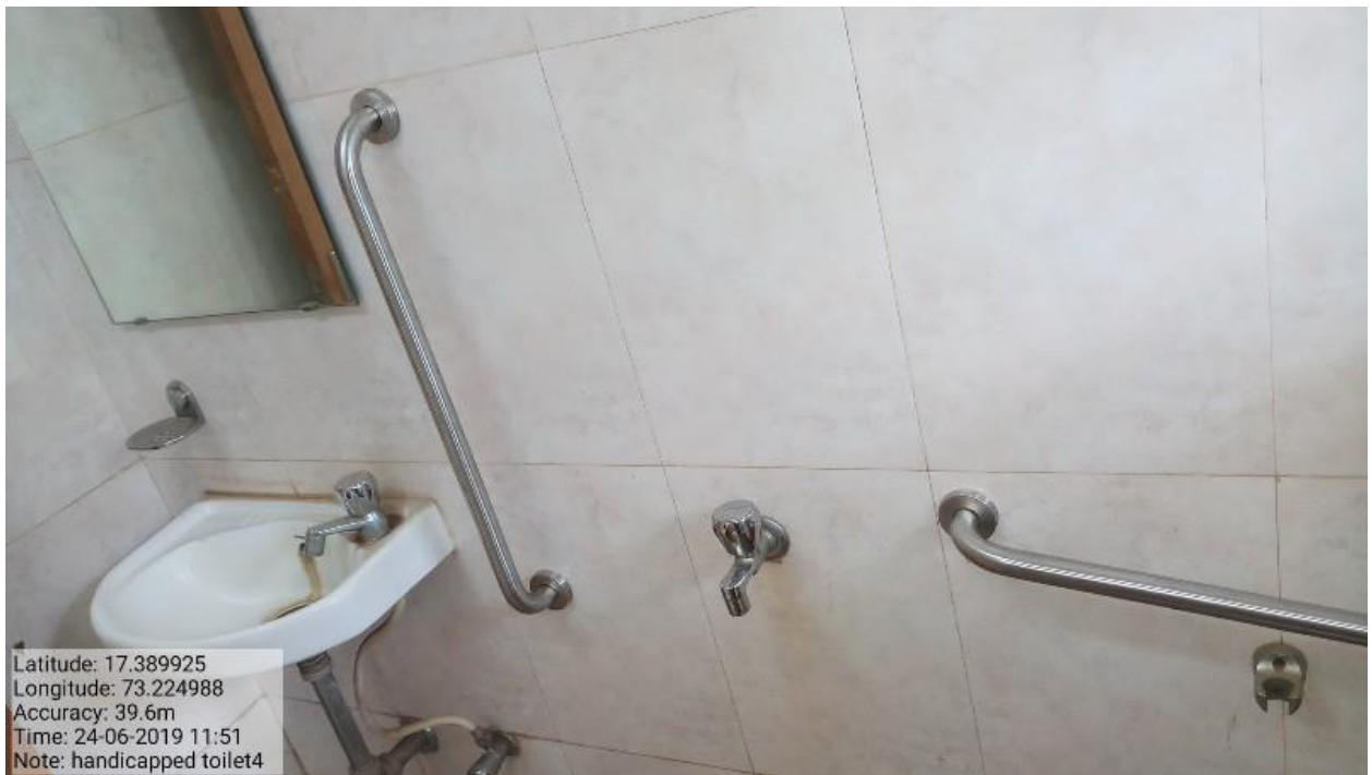
Special toilet for Handicapped students / staff with handle for support
