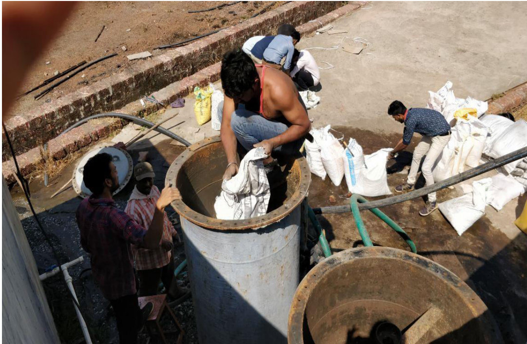
Replacement of filter media (22th March 2018)
