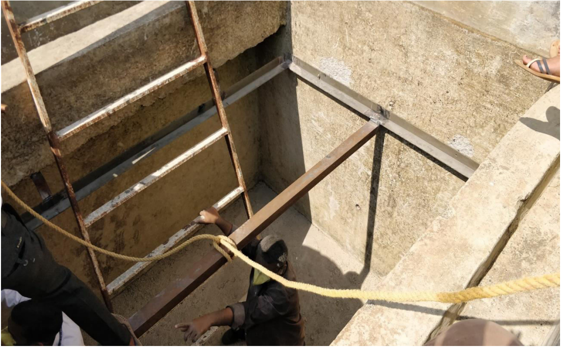
Installation of tube settler
