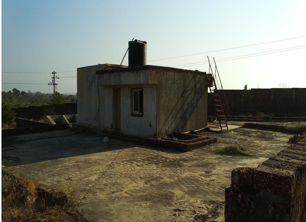
Sewage treatment plant at MPCOE campus
