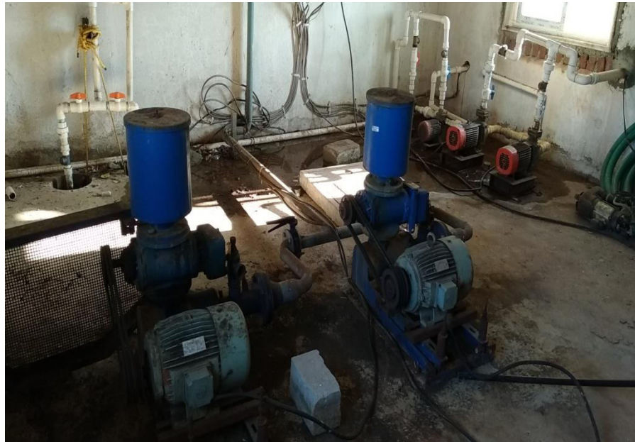
Compressed air blower, filter pump, feed pump assembly
