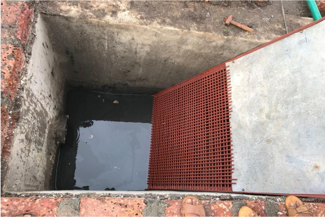
Installation of new bar screen
