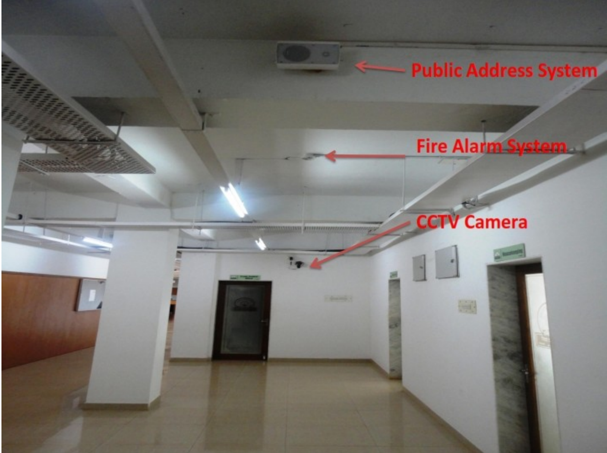
2.CCTV Strategic Location , Public Address System & Fire Alarm System.
