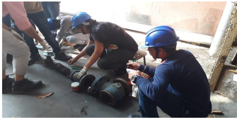
Students performing maintenance of valves
